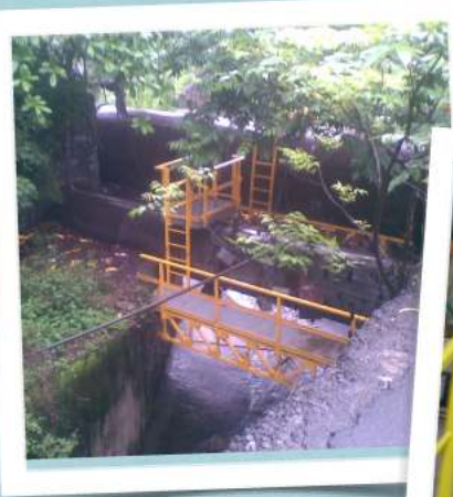
Ercon FRP/GRP Platform with Stair tread in a process plant.
