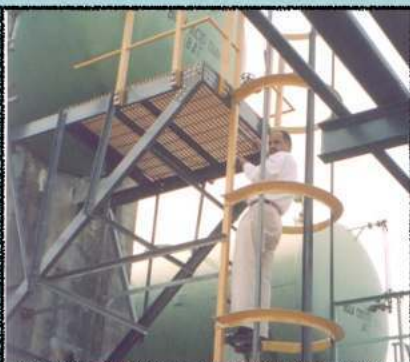
ERCON FRP Platform with Cage Ladder as approach to bulk acid storage tank in a refinery.
