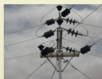
Cross Arm installed at Wind Mills site.
